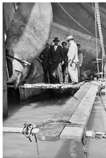
The faulty prop being removed, the stump of the missing blade clearly visible
