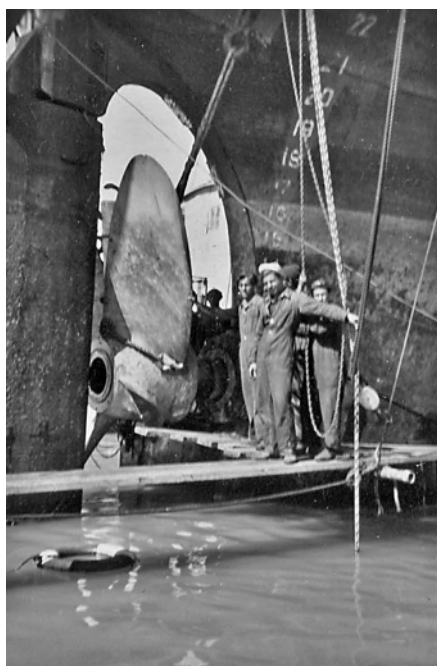
The faulty prop being removed, the stump of the missing blade clearly visible
