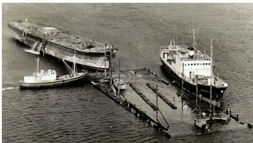
One of the attempts at docking.
