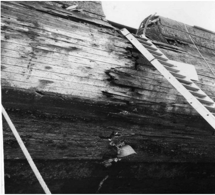
The crack, after it was closed up.
