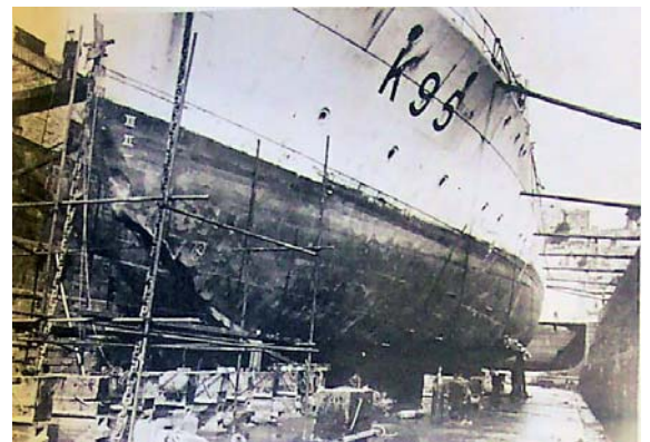
The damage sustained by Dianthus in the ramming of U.379
