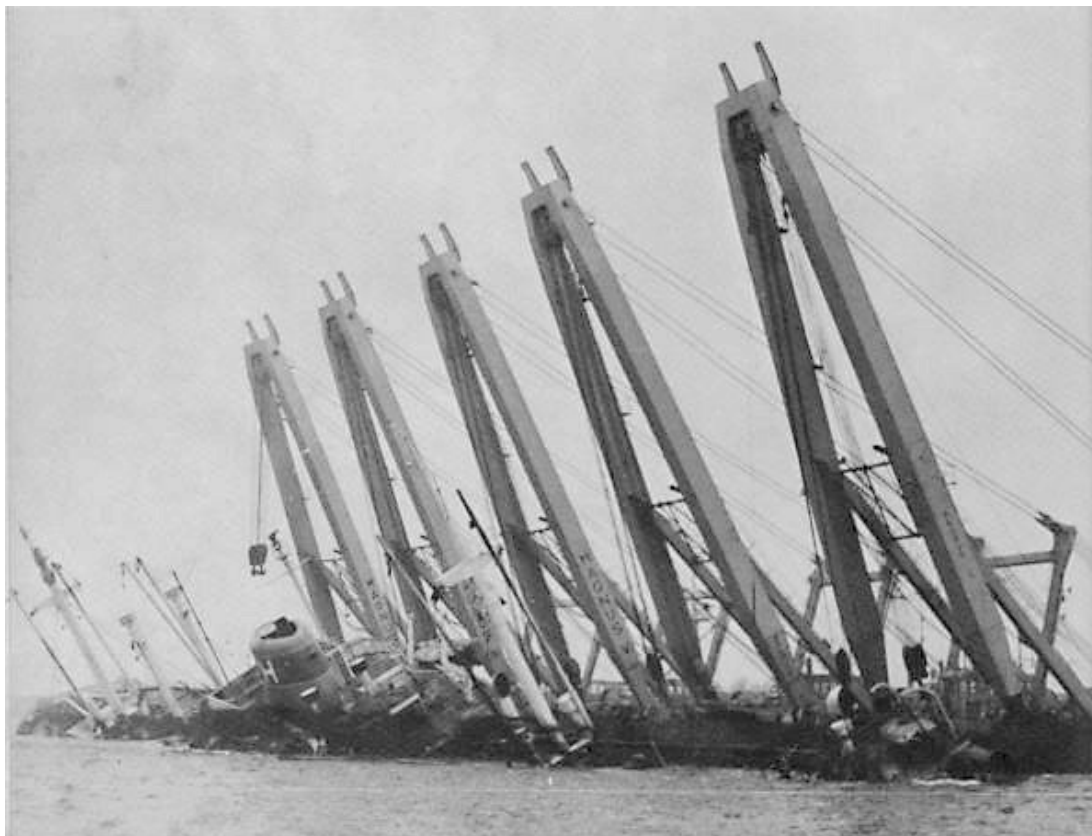
Parbuckling Hornland , Rotterdam Waterway 1969?
