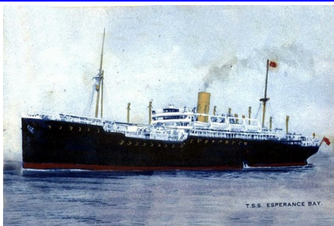
This particular class of Bay boats were twin screw ships of around 14,000grt and 531 ft long.
