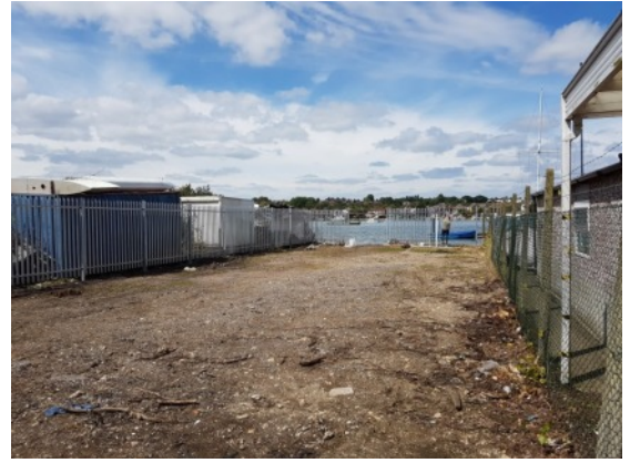
Fig. 2 - 14 August: Fencing makes the new site secure.
